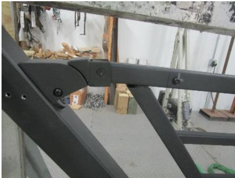
Photo No. 10 Stair Top Rail Bracket Connection
