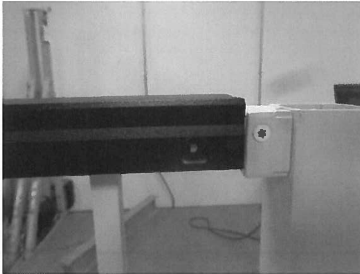
Photo No. 8 Rail Connection
