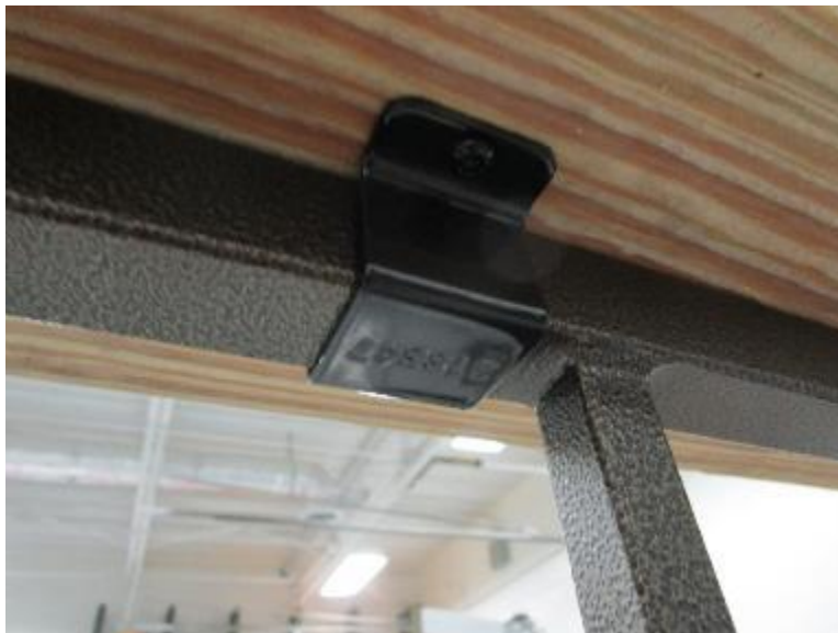
Photo No. 4 Wood Drink Rail Attachment Bracket
